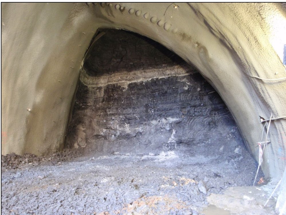
Figure 4: Tunnel face with thick bedding through the excavation
