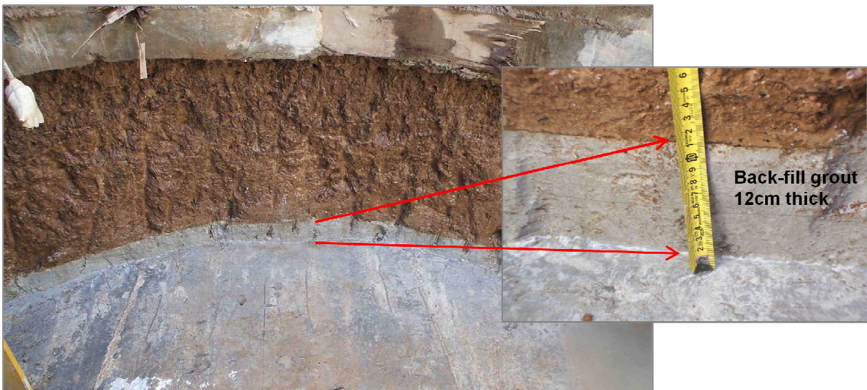
Figures 7. The image shows the hardened grout after removing the ground above the short tunnel.
