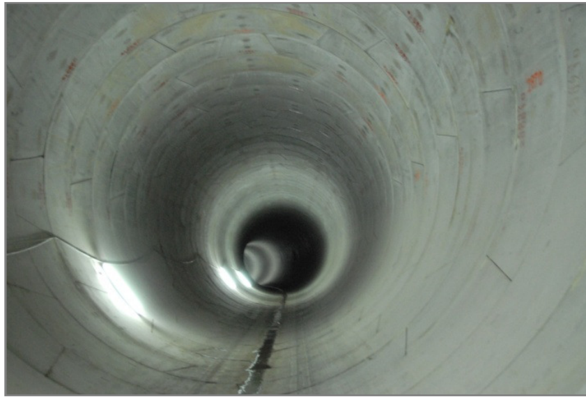
Figure 2. The completed short tunnel
