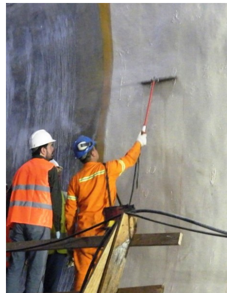
Figure 10: High voltage holiday testing to confirm integrity of membrane
