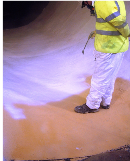
Figure 4: spraying membrane to invert
