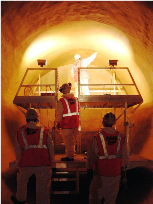
Figure 1: access platform enabling application to 360° of the tunnel
