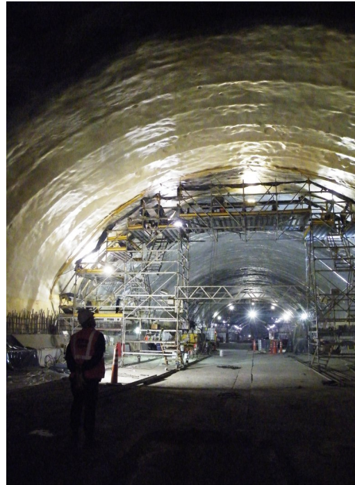
Figure 2: system scaffold providing access from multiple platforms
