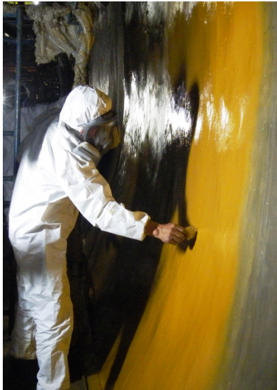
Figure 3: wet film thickness testing during spraying
