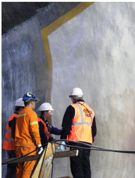
Figure 9: tidy edge terminations facilitate clean, effective laps
