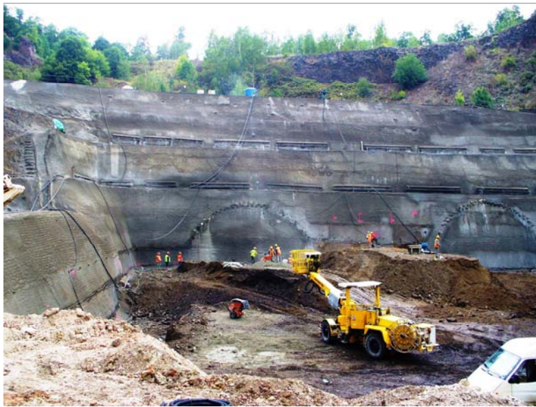
Fig. 3 Prague's portal area prior start of tunnel excavation
