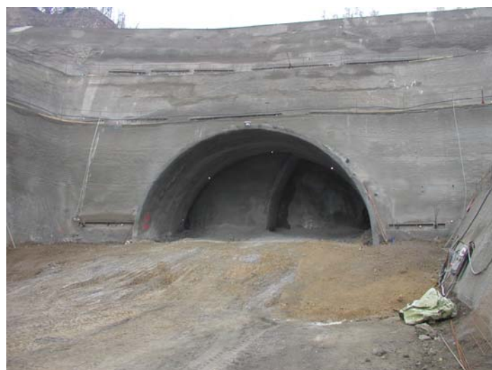
Fig. 4 Excavation with splitted top heading
