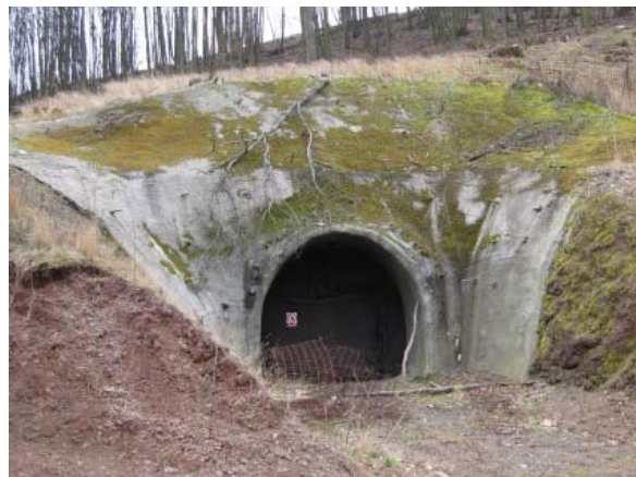
Fig. 2 The exploratory gallery excavated in advance
