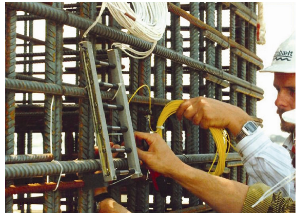
Fig. 6 Preparing embedded corrosion sensors for monitoring of reinforcement
