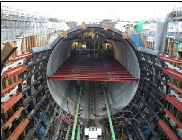
Figure 9. Temporary strut installing
