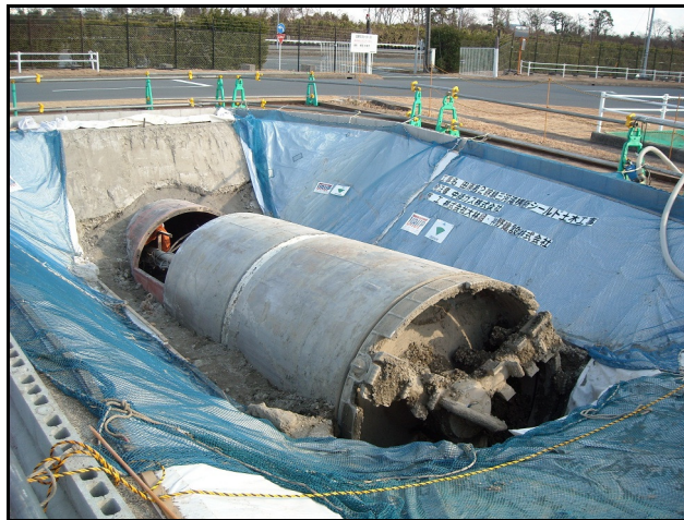
Figure 14. TBM arrival
