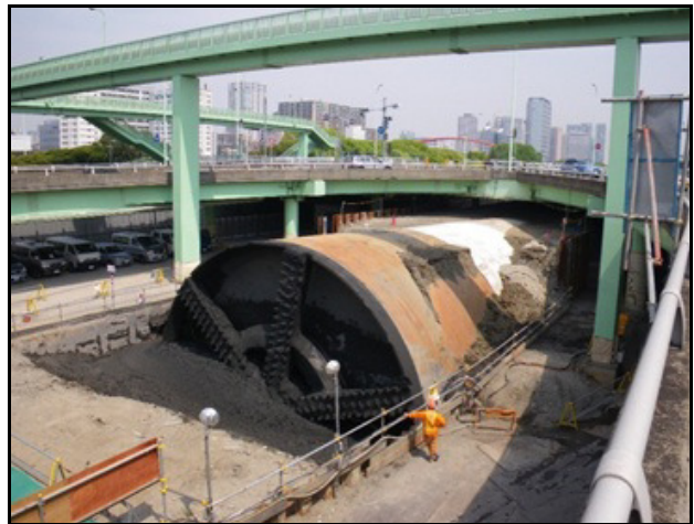
Figure 10. TBM arrival
