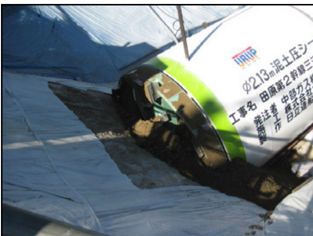
Figure 12. TBM launching
