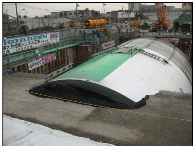
Figure 8. TBM launching
