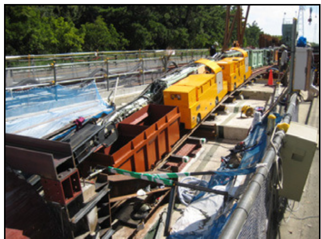
Figure 13. TBM trailing gears
