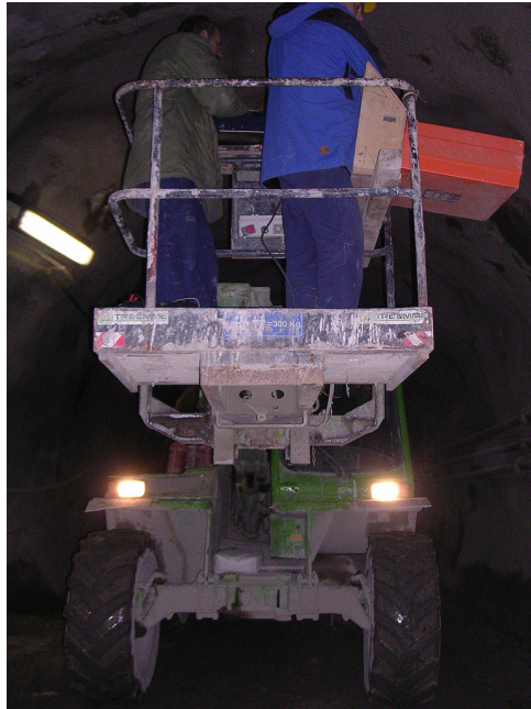
Fig. 2. GPR measurements in the tunnel
