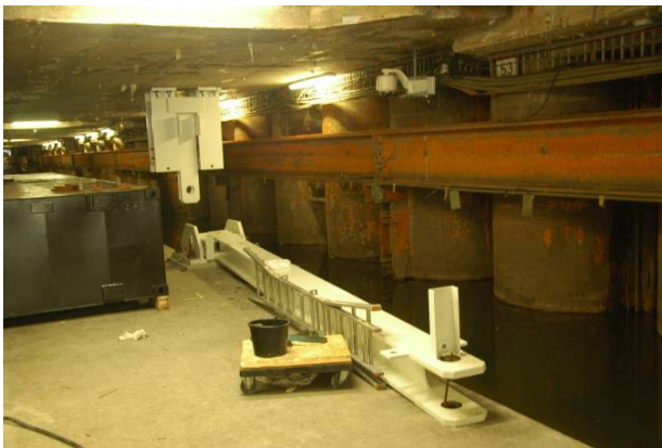
Fig. 8 Suspension beams on tunnel deck
