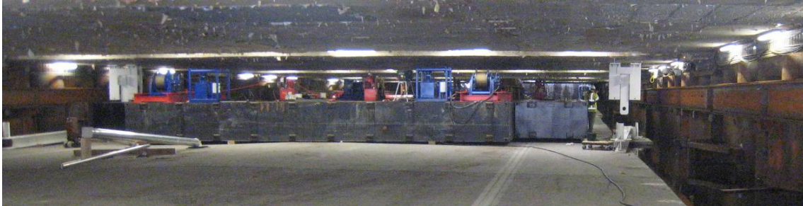
Fig. 5 TE and pontoons under roof slab
