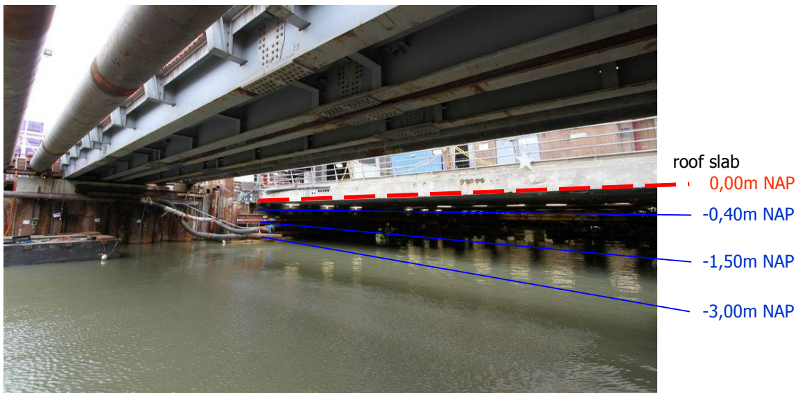
Fig. 3 Water levels in immersion trench
