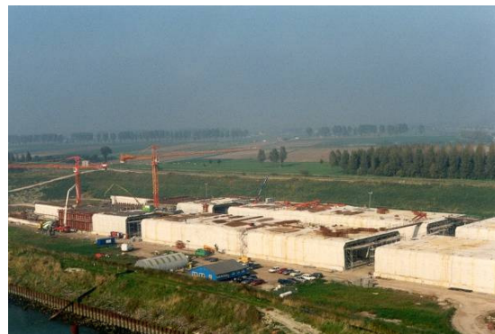
Fig. 2 Construction dock in Barendrecht (Wijkertunnel)
