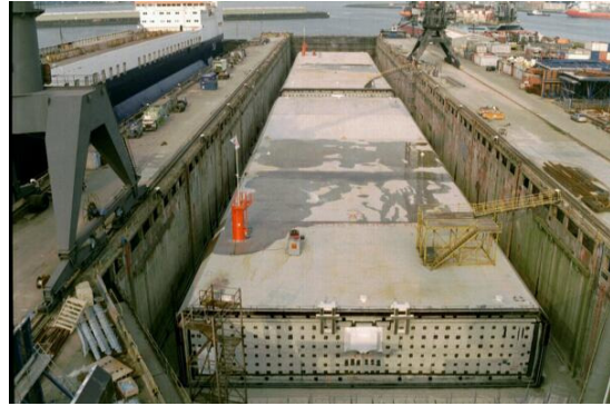
Fig. 4 Construction in a ship dock (Calandtunnel)
