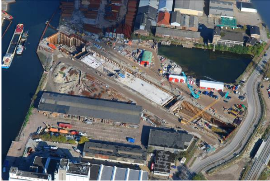
Fig. 3 Construction dock in the approach of the tunnel (N57)
