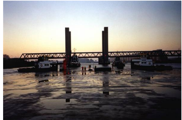
Fig. 11 Passage of a bridge (Calandtunnel)
