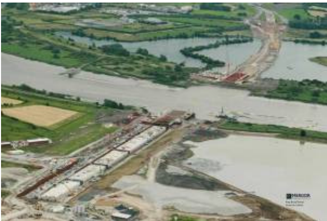
Fig. 21 Overview Shannon tunnel (Limerick, Ireland)
