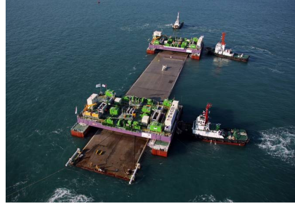
Fig. 15 Immersion with pontoons (BGFL, Korea)
