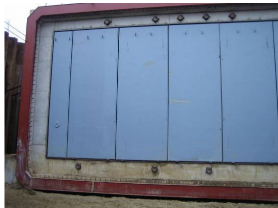
Fig. 5 Steel bulkhead (Roertunnel, Netherlands)
