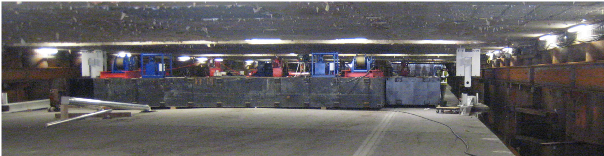
Fig. 32. TE and pontoons under roof slab (NS-line, Amsterdam)
