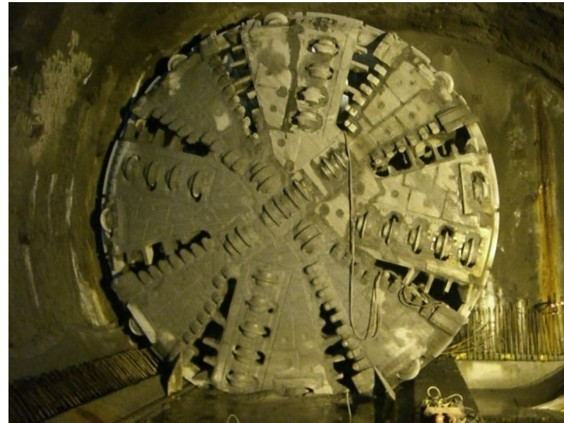
TBM-360 cutting head with grizzly bars
