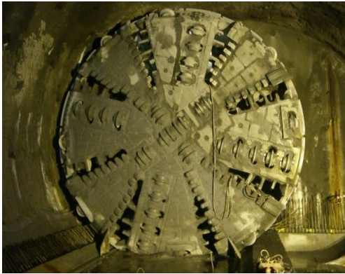
Putting grizzly bars on cutterhead
